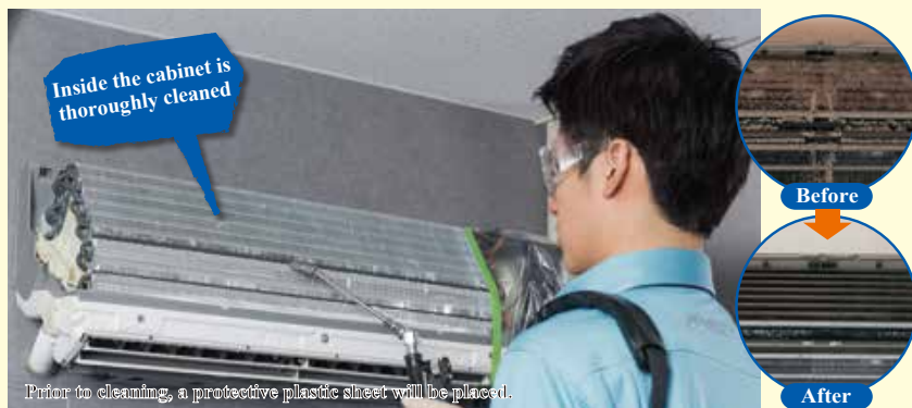
Prior to cleaning, a protective plastic sheet will be placed.
