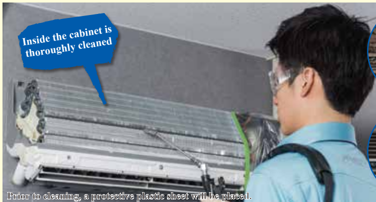
Prior to cleaning, a protective plastic sheet will be placed.
